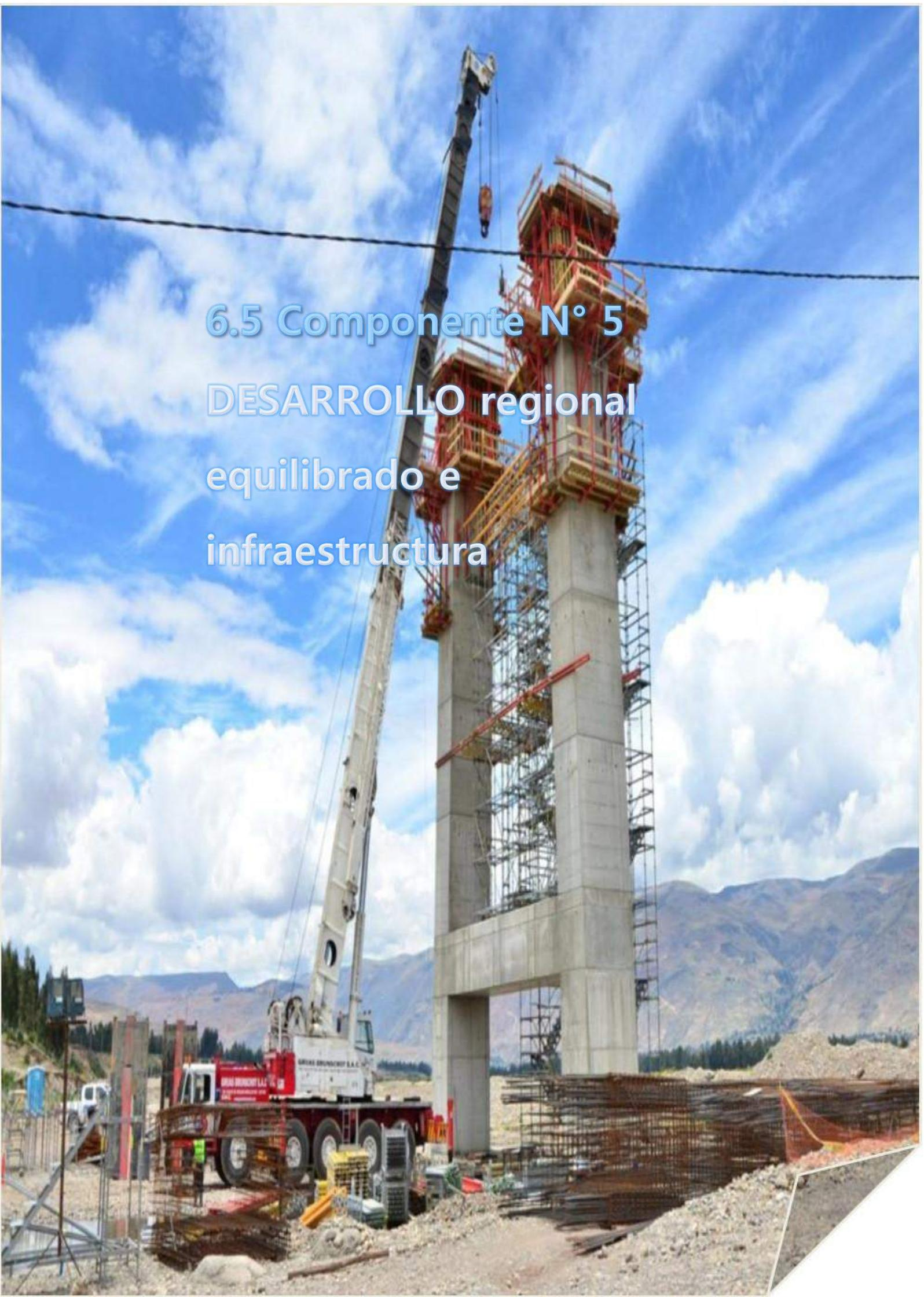
A tall, rectangular concrete bridge pier is under construction. The pier is surrounded by extensive scaffolding and wooden formwork. A large white crane with a red base is positioned at the base of the pier, with its boom extending high up. The background shows a clear blue sky with scattered white clouds and distant mountains. The ground is a mix of dirt and gravel, with some construction materials and equipment visible.
